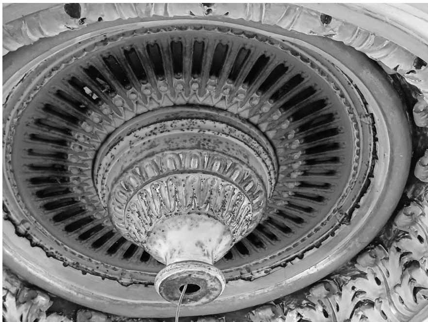
Detail of the ceiling at Bryn Sion Baptist Chapel, Mill Street, Trecynon, Aberdare (photograph copyright National Churches Trust)
