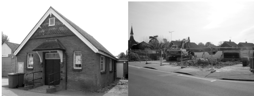
Primitive Methodist Mission Room (1885), Rushams Road, Horsham, West Sussex: seen (left) in June 2010 and (right) in April 2018 immediately after demolition. Holy Trinity Church is just visible on the right (photographs copyright Matt Davis)
