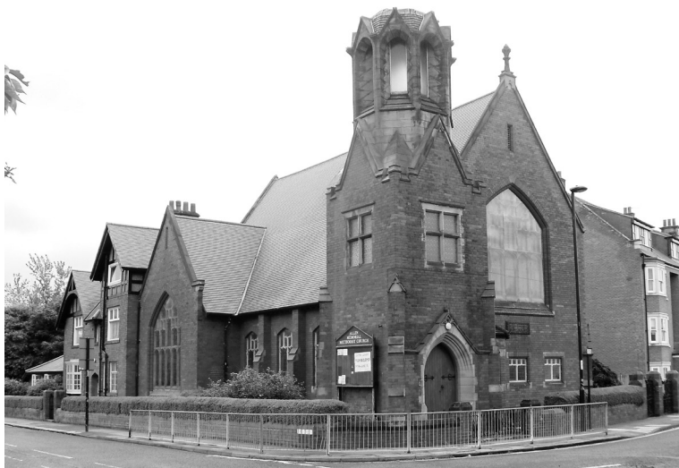
The Allen Memorial Methodist [New Connexion] Church in 2010, showing the stub of the stone steeple (photograph copyright Bill Henderson, adapted from geograph.org.uk/photo/2989344 : licensed for reuse under Creative Commons licence CC BY-SA 2.0)
