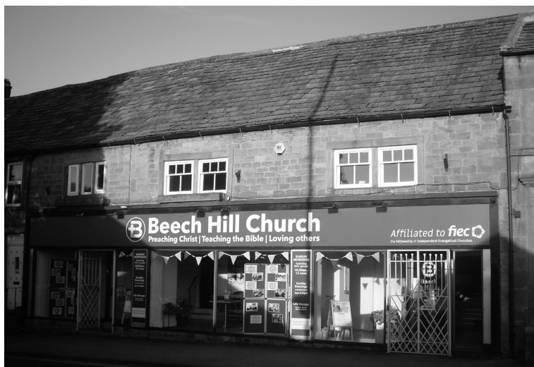
The new Beech Hill Church in July 2022; note the prominent FIEC branding (photograph copyright Gerard Charmley)
