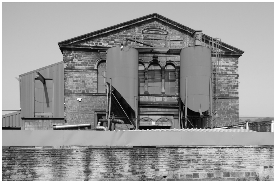
The former Wesleyan Methodist Church, Dalton Lane, Keighley, West Yorkshire, seen in September 2023. The date-stone is partly hidden behind the metalwork (photograph copyright Kenneth Jackson)
