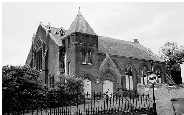
The former St Clement's Congregational Church, Ipswich, seen in May 2022.
