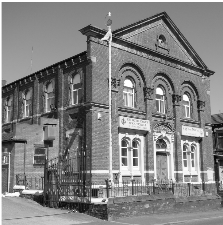
Sri Guru Nanak Sikh Temple, Tong Road, Leeds (formerly Mount Pisgah Methodist Chapel), seen in April 2023; its origins as a United Methodist Free Church are clear from the lettering below the pediment. Note also the Sikhs' traditional orange flagpole (photograph copyright D. Colin Dews)
