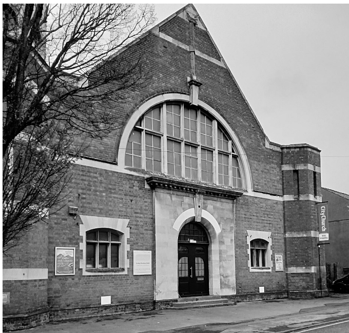
The main (east) elevation of the chapel in November 2022, showing the Portland stone door surround (photograph copyright Ian Serjeant)
