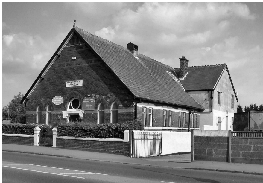
The former Clegg's Lane Methodist Church, Little Hulton, Greater Manchester, seen in 2010.
