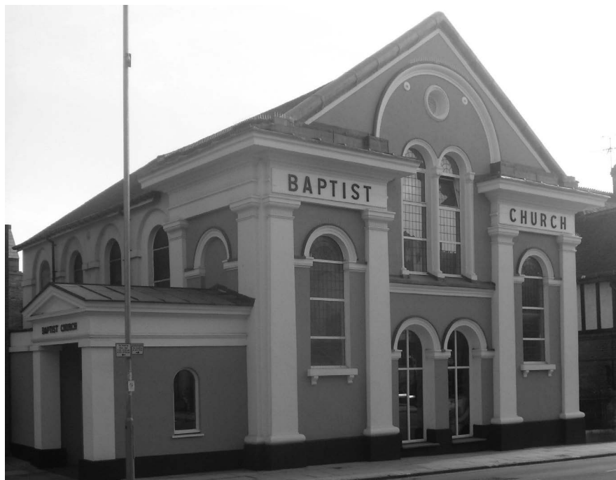
Winchester Baptist Church, City Road, Winchester, in May 2021. The tunnel-like porch on the left is to be replaced by a striking glass box (photograph copyright Matt Davis)
