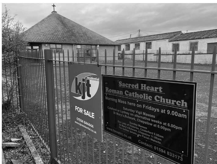
Church for sale: the former Church of the Sacred Heart (1988–2018), Sedbury, Gloucestershire, in December 2021, by which time planning permission had already been granted to convert the interior into flats. The wartime hut in the background was the original church, dedicated in 1939 (photograph by Alan Hughes, adapted from geograph.org.uk/photo/7042626 ; licensed for reuse under Creative Commons licence CC BY-SA 2.0)
