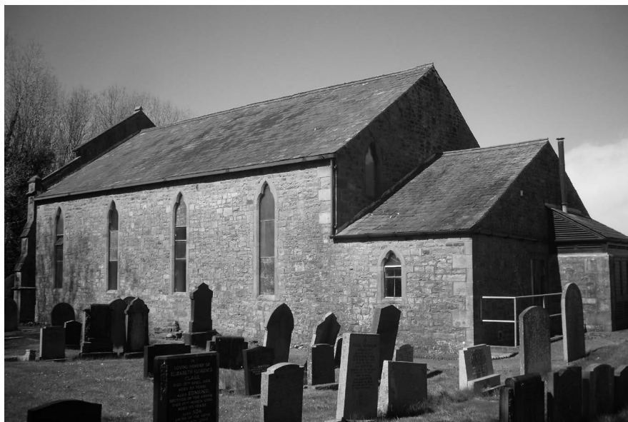
The side and rear elevations of the chapel in April 2021, also showing part of the graveyard (photograph copyright Gerard Charmley)
