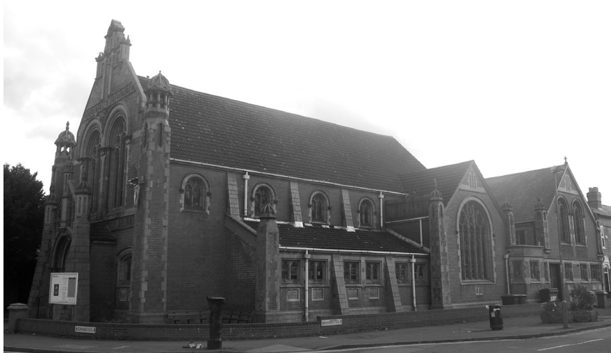
Turn-of-the-century terracotta: the Grade II-listed Edward Road Baptist Church, Balsall Heath, Birmingham, seen here in March 2022, features bold and intricate buff terracotta decoration. The chapel dates from 1899; the schoolrooms to the right were added in 1900 (photograph copyright Matt Davis)
