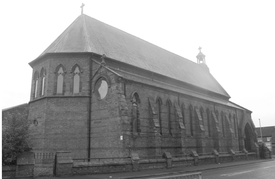
The former St Marie's Church, Newtown, Widnes, photographed in September 2021
